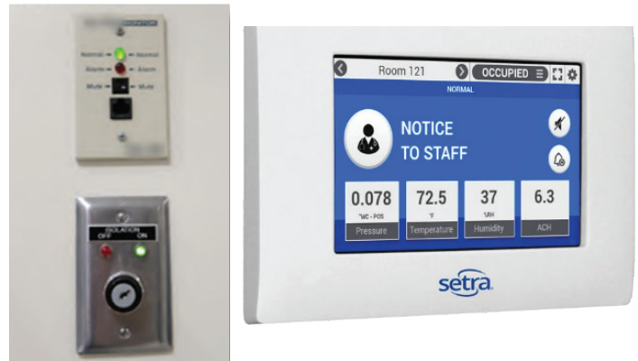
Images 8 and 9. Negative pressure room monitors (left: Cal/OSHA; right: SETRA)
